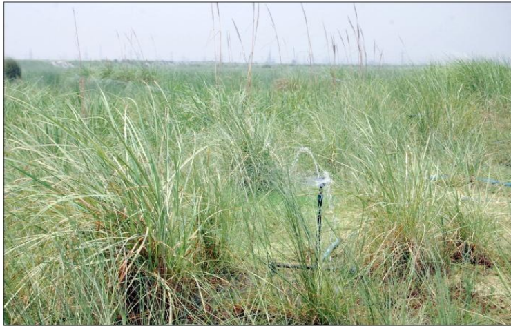
Sprinkling System at ash dyke Units 1to 6 of PTPS
