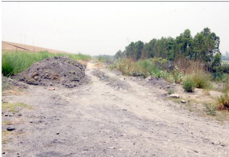
Plantation along with Ash dyke Units 7&8 PTPS
